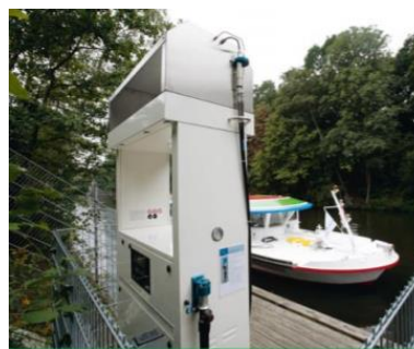
Figure 117 GH 2 dispenser at the pier. [136]
