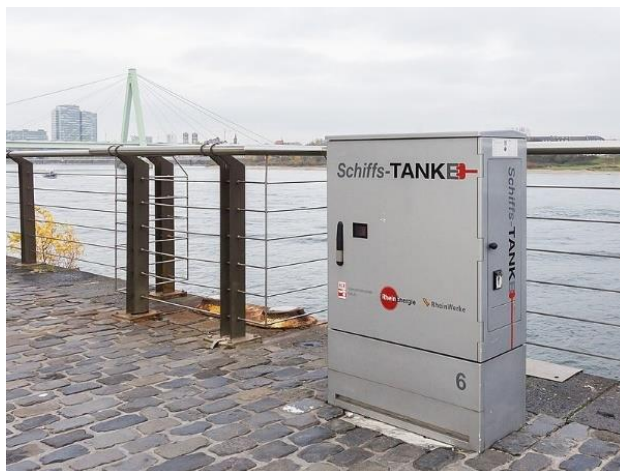
Figure 113 Shore power supply at the Rheinauhafen in Cologne. [160]
