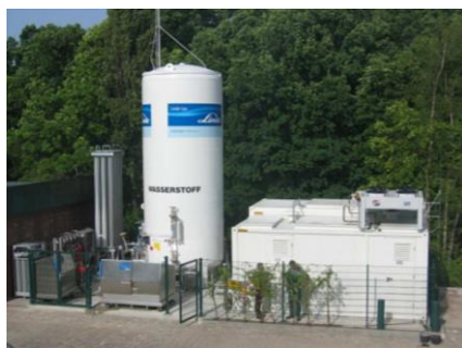
Figure 116 H 2 -liquid hydrogen tank with compressor and buffer tank. [137]
